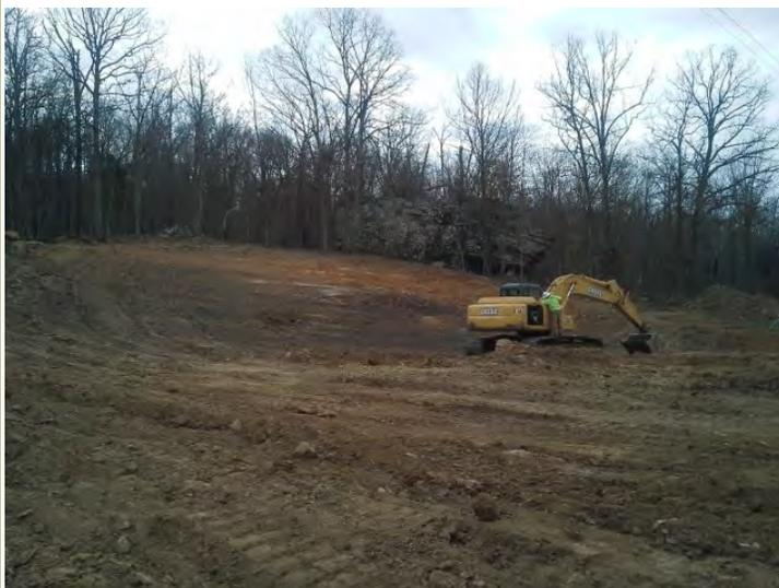
Work has begun at the Water Treatment Plant with the general Contractor J.L. Bryson getting a large area cleared for the new chemical building. Last week footings were poured as well as the slab for the new building. The contractor will focus on work that does not effect current treatment first then shift gears to work that
